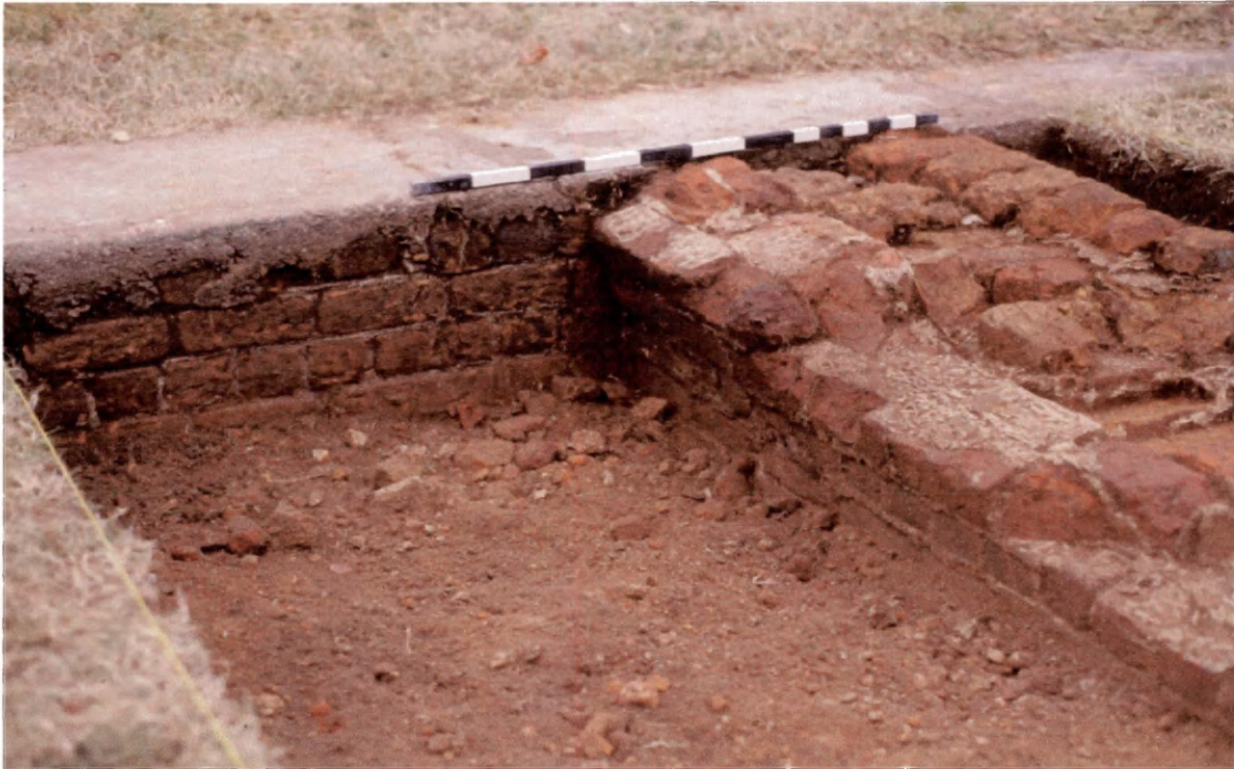
Springer course forming the arching base of the brick vault in the cellar. Courtesy of the Colonial Williamsburg Foundation.
